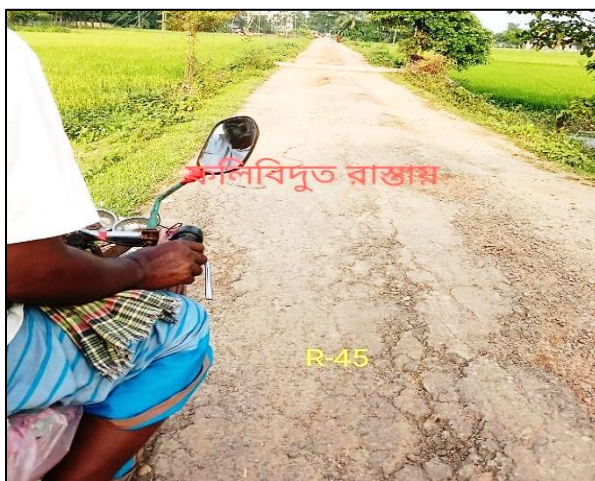
R-45 Improvement of Road by BC to RCC from Pollibiddut Sub - station towards Jahangirpur Fazil Madrasa (Ch. 0.00m to Ch. 805m) & installation of Street Light 28 nos. at ward no. - 07, Madan Paurashava, Netrokona. Total Length = 805m.
